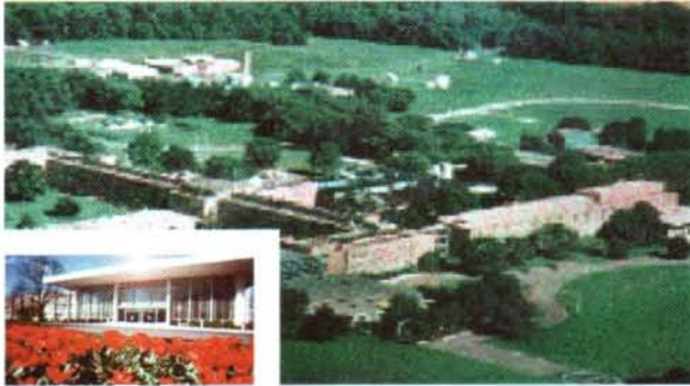
The David Sarnoff Research Center in Princeton, New Jersey, is one of the world's leading R&D facilities
